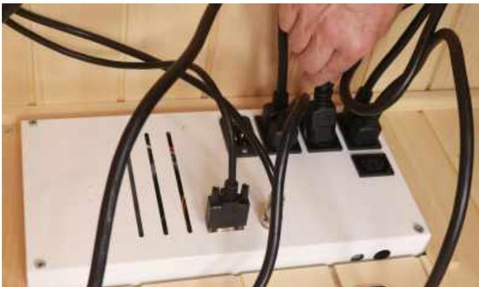
Plug in all heater leads to receptacles in the power supply box.
