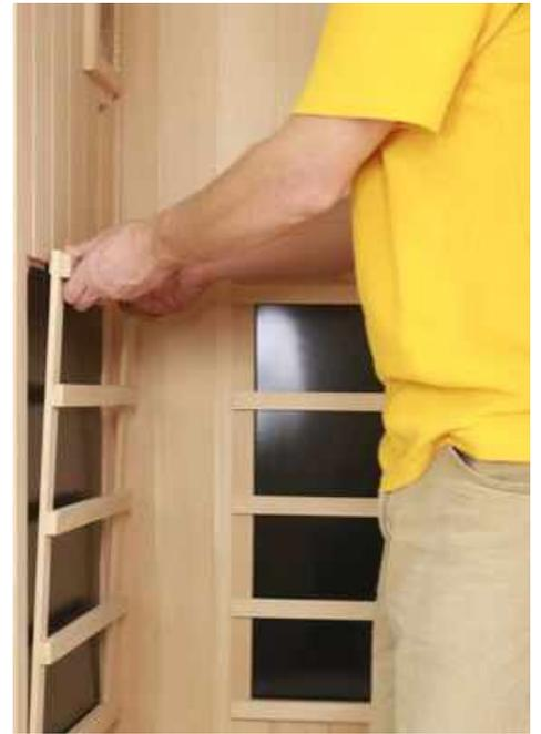
Reinstall the side wall heater guards
