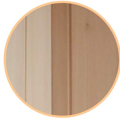
There are two sets of fasteners to join the saunas' corners together. After lowering the Side Wall, check to ensure that both sets of fasteners have connected by looking at the corner inside of the sauna. It is possible to connect one set of fasteners and miss the other. If there is an obvious gap in the corner between the two walls at least one fastener has not connected and the raising and lowering procedure will need to be repeated.
