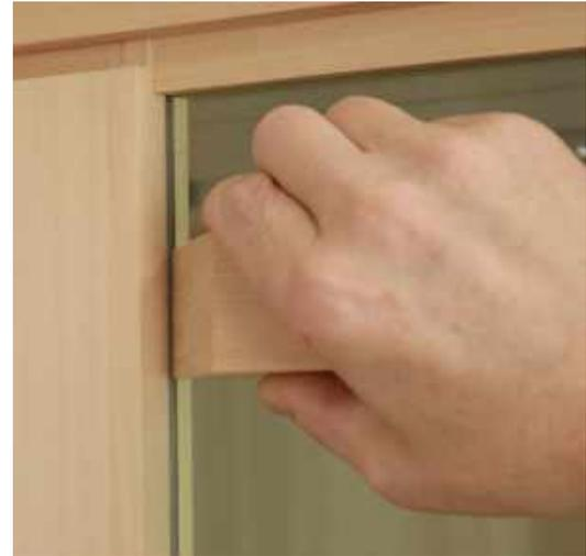
Small wooden block (included) can be used to fully press the glazing strip into channel
