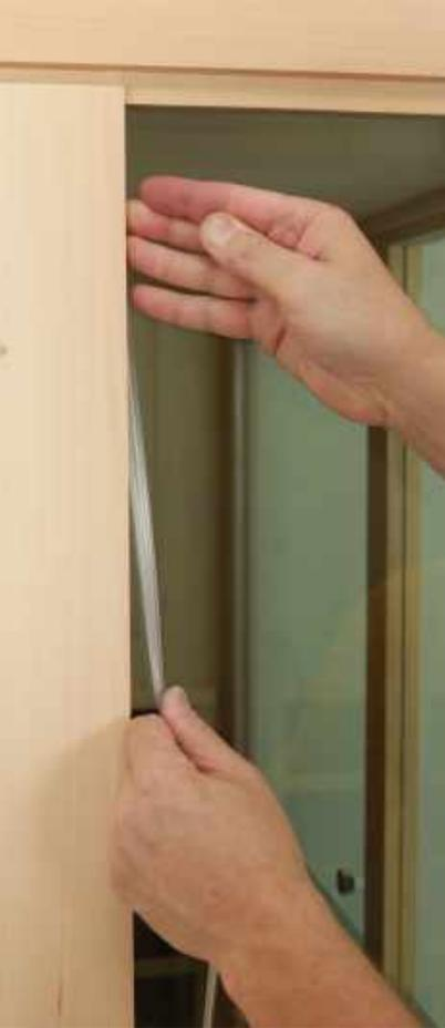
Firmly press flexible glazing strip into wood channels along the outside of the Side and Front Wall glass panels.
