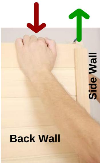
Cinch the Left Side Wall and the Back Wall together by applying pressure on the outside of the Left Side wall.
