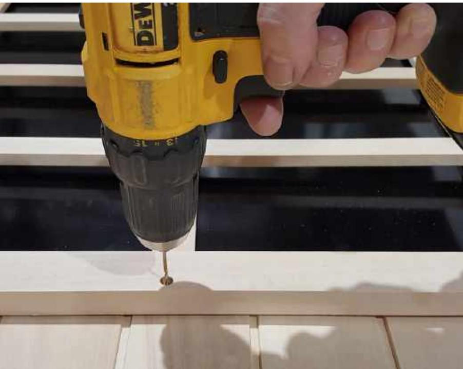
Drill a pilot hole into the wall through the holes in the heater guards. Do not drill deeper than necessary for the length of the screw.
