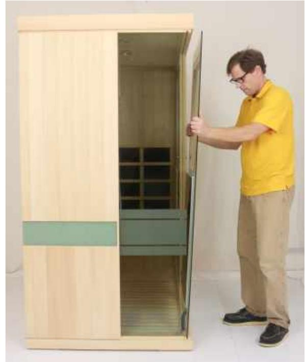
Carefully insert the bottom edge of the Front Wall glass panel into the slot in the Floor base. The Front Wall glass panel must be positioned so that the heater panel is fitting inside of the Side Wall glass panel.
