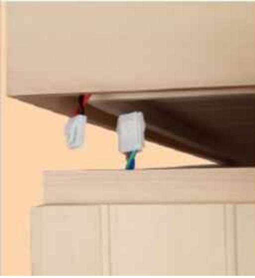
Connect the 12 Volt power supply wire at the back left corner of the sauna.
