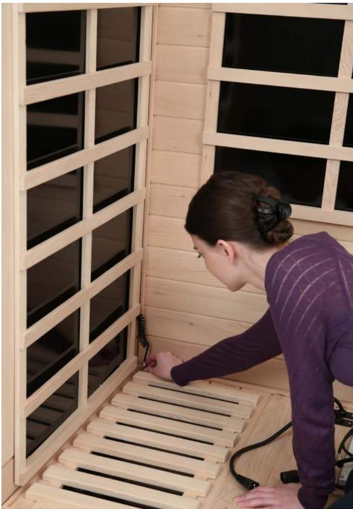
**Connect the Front Wall heater electrical lead to the floor base.**
