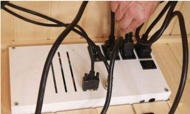
Plug in all heater leads to the receptacles in the Power Supply Box.
