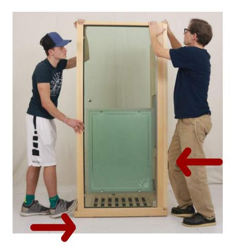
**Connect Side & Front Wall** Cinch the two walls together by applying pressure on the outside of the side wall with your knee
