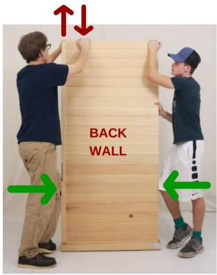
Repeat procedure to connect the Back Wall to the Right Side Wall. Raise the side wall up approx 3/4". NOTE: Do not raise the Side Wall any further than necessary. Raising the Side Wall too much may disrupt the connected front corner
