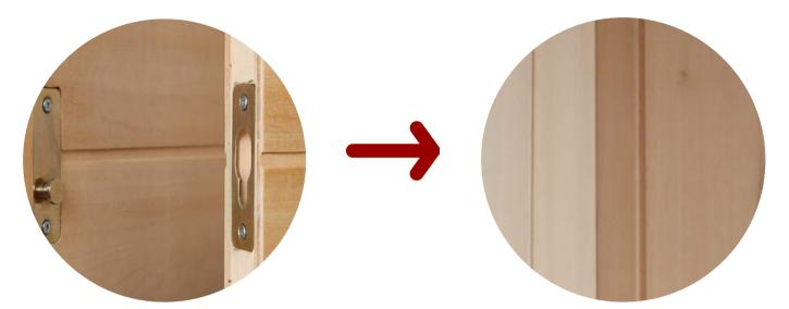
Check to ensure that both sets of fasteners have connected by looking at the corner inside of the sauna. It is possible to connect one set of fasteners and miss the other. If there is an obvious gap in the corner between the two walls the fasteners have not connected and the raising and lowering procedure will need to be repeated.
