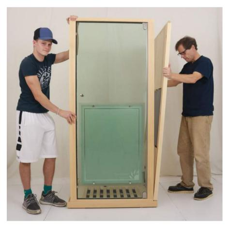
**Position Right Side Wall** Lift the Right Side Wall into position wedging the bottom of the wall into the channel in the floor base.
