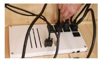
Plug in all heater leads to the receptacles on top of the power supply box.
