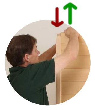
Slide the Back Wall up approx. 3/4" while holding the Side Wall down with your opposite hand. The 2 sets of fasteners for the walls will connect when the back wall is raised sufficiently. When you feel the fasteners connect, slide the Back Wall back down.
