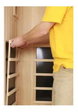
Reinstall the side wall heater guards
