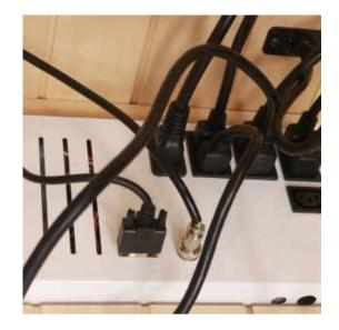
Feed the main power supply cord in through the hole in Back Wall and insert in power supply box. Do NOT plug power cord into your wall outlet until all electrical connections are finished inside of the sauna.
